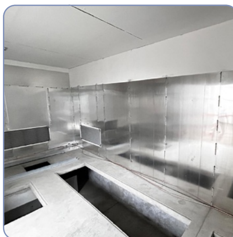
Cabina ente distributore - Torino (TO) Distributor cabin - Turin (TO)
