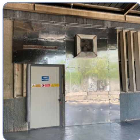
Capannone industriale - Pisogne (BS) Industrial warehouse - Pisogne (BS)
